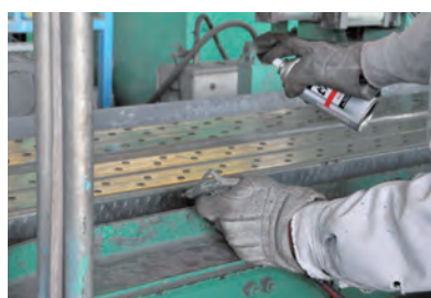
Anti-rust repair for scaffolding of construction
